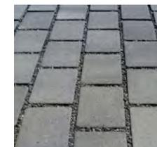
Figure 328. Examples of permeable paving materials.
