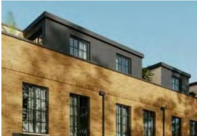
Figure 212. Flat roof with the top floor set back.
